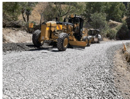
Pavement Work – Route 52
