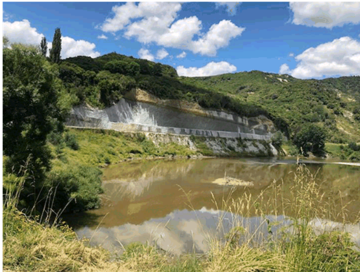
Photo: Taken standing on the August 2018 Jerusalem dropout, looking over to the June 2015 completed repair
