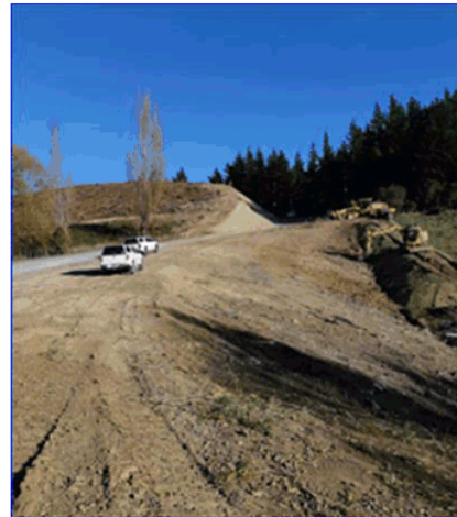
Route 52, 63 Section – Large Road Realignment
